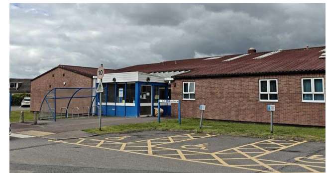
Western aspect of building B1
