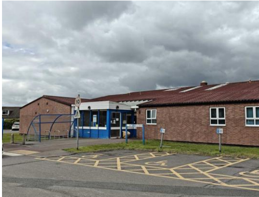
Eastern aspect of building B1
