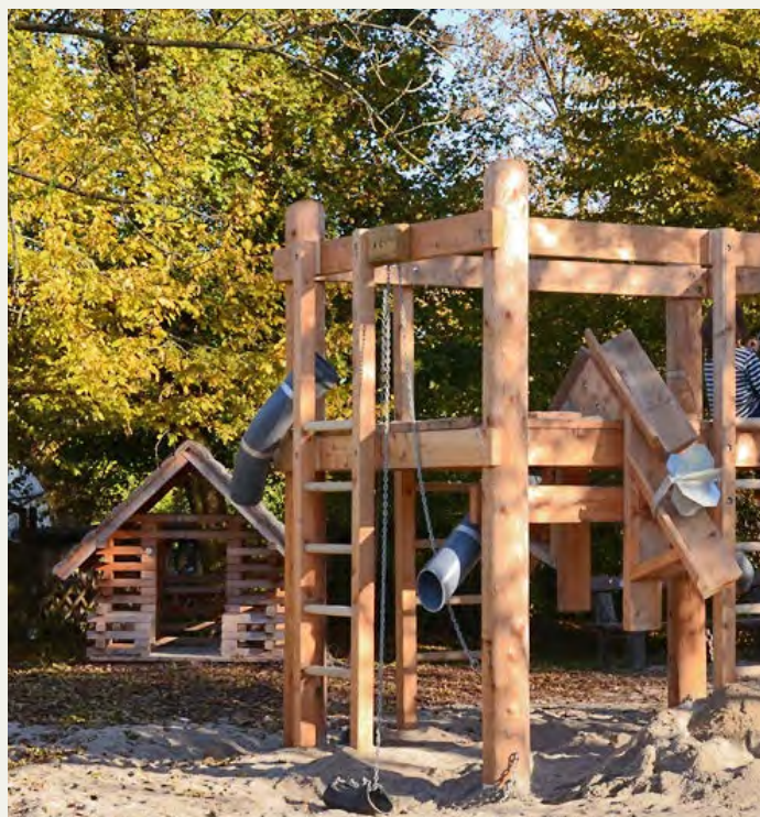
Timberplay Building Site
