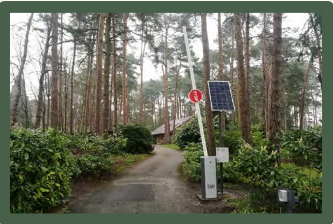
Automated barrier controlled entrances with number plate recognition cameras recording entry and exit times. Parking will be charged at the same rates as those at Staunton Water and Havant Thicket car parks.
