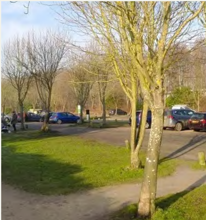
Tarmac broken out for Tree Planting
