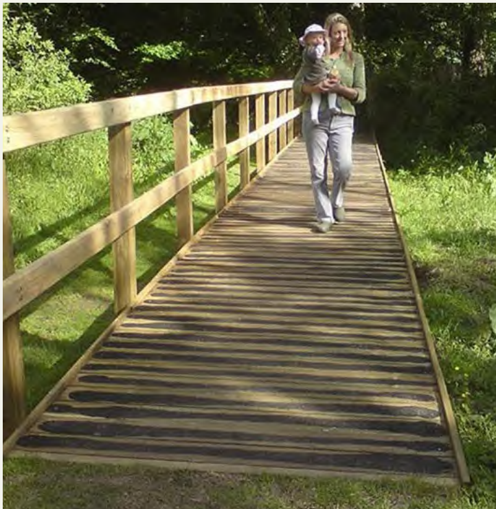
FSC sourced timber boards
