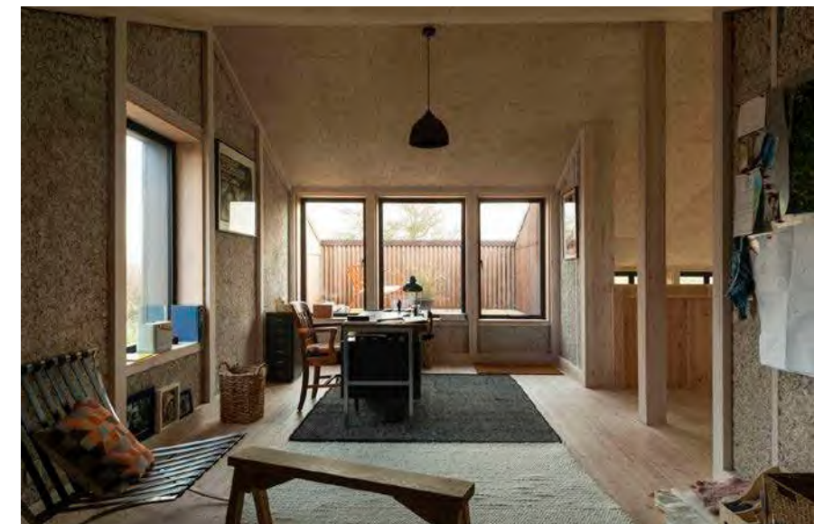
Hempcrete cassettes used at Flat House by Practice Architecture
