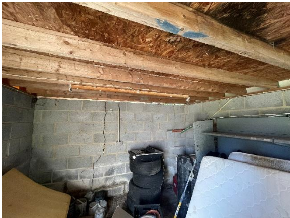
Photo 7 – Internal view of building 4.
