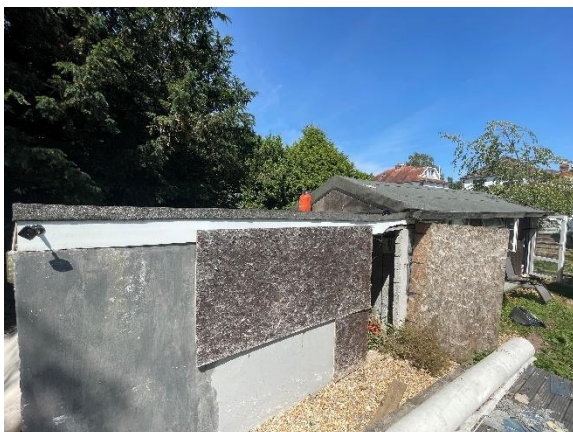
Photo 5 – Building 3 & 4 within the garden curtilage.
