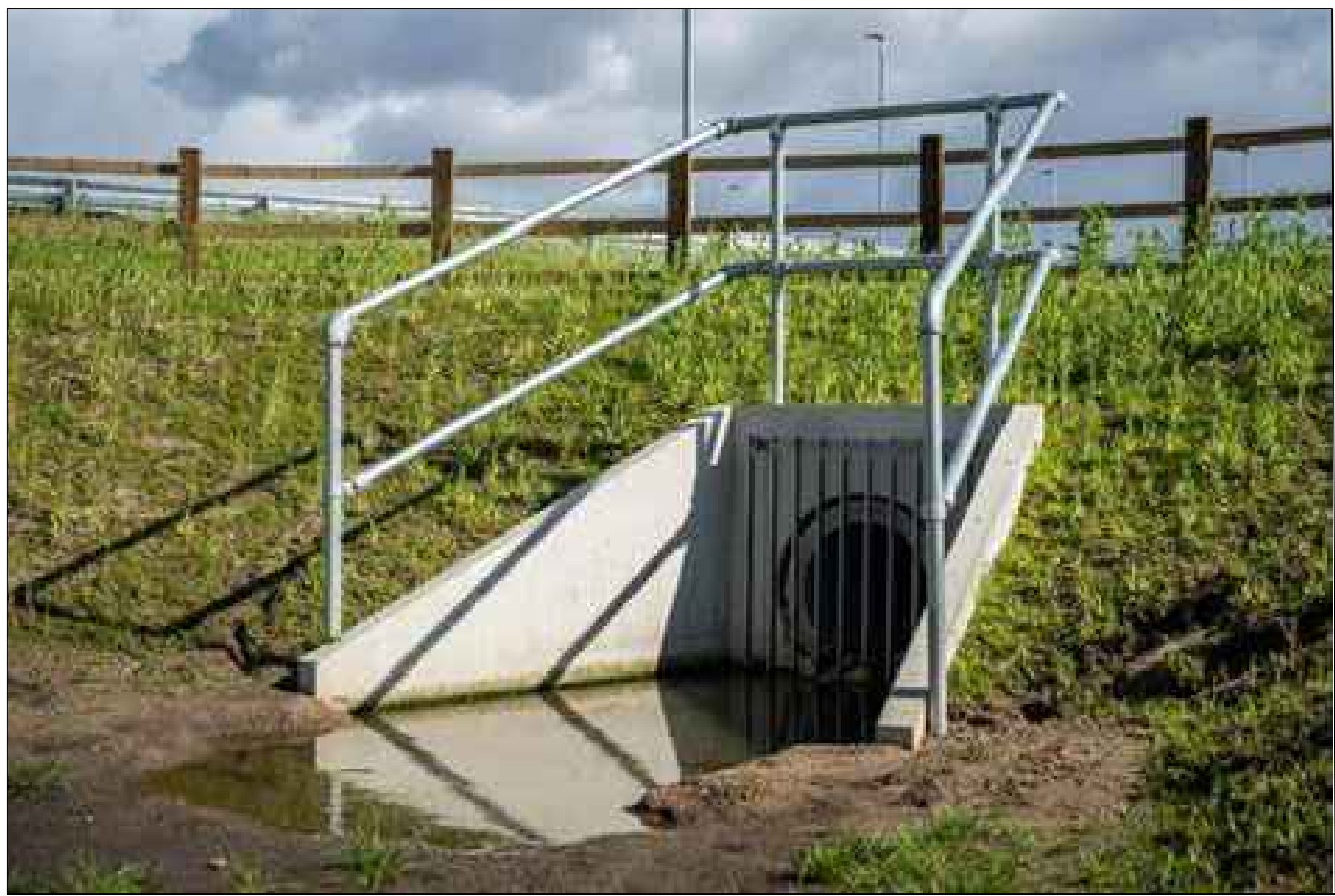
TYPICAL HEADWALL (ALTHON OR SIMILAR):
