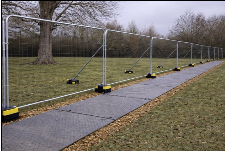
Ground protection example — woodchip and trackmats
