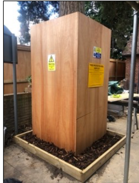
Trunk Protecta® ( GreenGridSystems.com ) & Timber stem protection boxing
