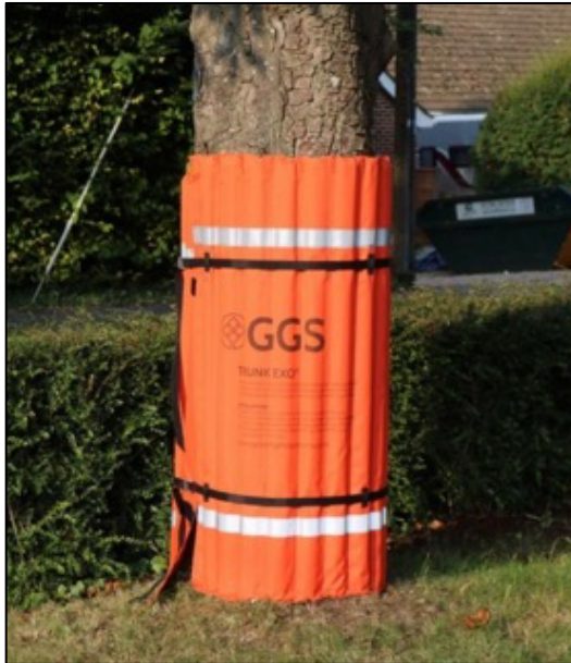
Trunk Protecta® ( GreenGridSystems.com ) & Timber stem protection boxing
