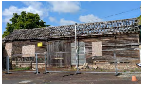
Photo 17. Eastern elevation of B7
