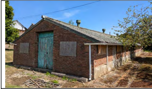
Photo 33. Western and southern elevations of B13
