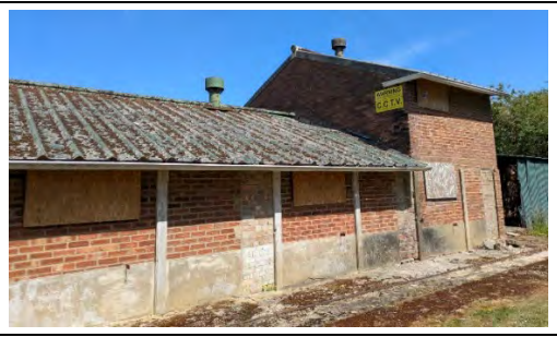
Photo 34. Southern elevation of B13
