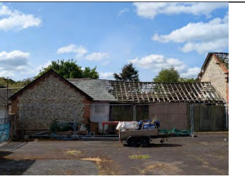
Photo 24. Northern elevation of B10
