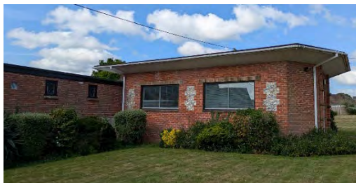
Photo 15. Eastern and northern elevations of B6
