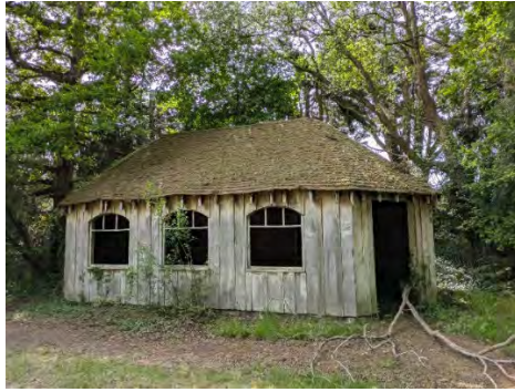
Photo 9. Eastern and northern elevations of B4
