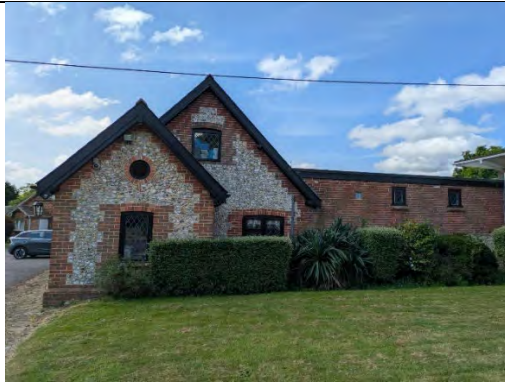
Photo 11. Northern elevation of B5
