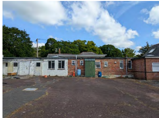
Photo 14. Southern elevation of B6
