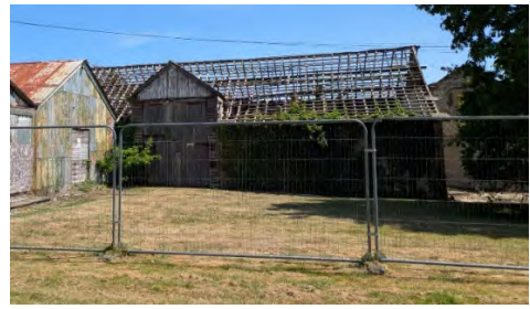
Photo 18. Western elevation of B7 (centre of image) and southern elevation of B8 (left of image)
