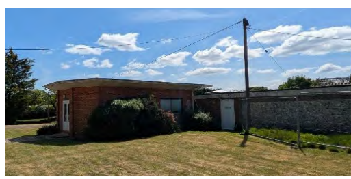
Photo 16. Western and northern elevations of B6
