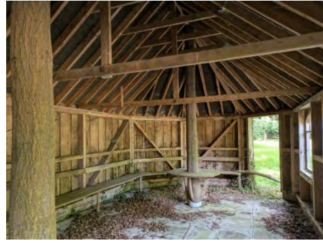
Photo 10. Internal view of B4
