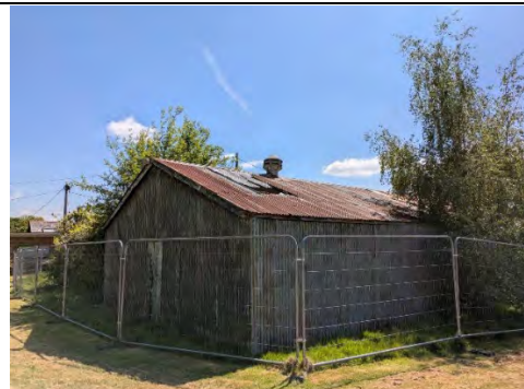
Photo 22. Northern and western elevation of B9
