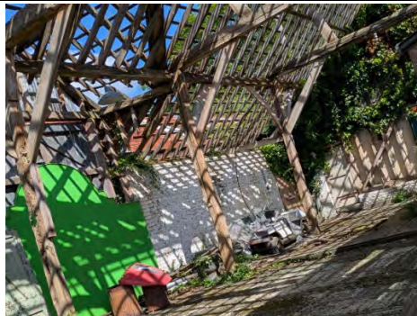
Photo 19. Internal view of B7
