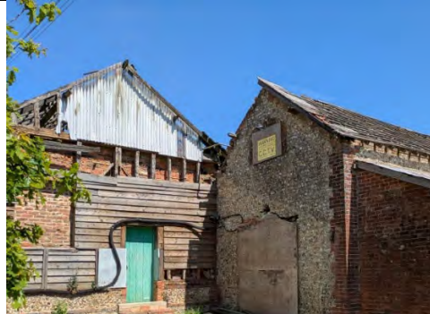
Photo 20. Southern elevation of B7 (left of image) and western elevation of B10 (right of image)
