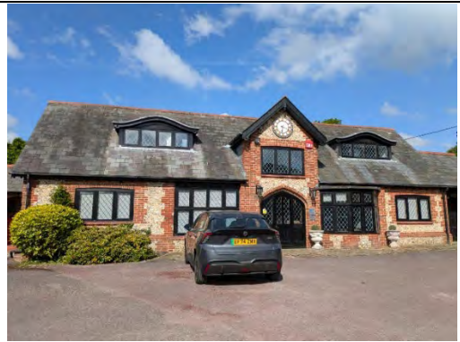
Photo 12. Eastern elevation of B5
