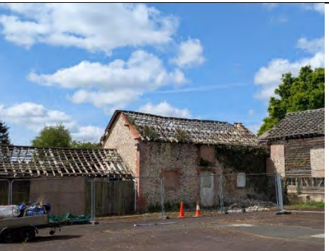
Photo 23. Northern and eastern elevations of B10 (centre of image) and eastern elevation of B7 (right of image)
