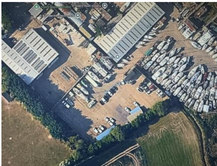
Aerial context of the Top Yard and adjoining fields
