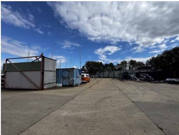
Photograph 4B Additional view within the Top Yard 11 September 2026
