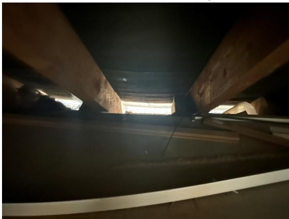
Photo 3 – Light leaks and access point within the void space of building 1.
