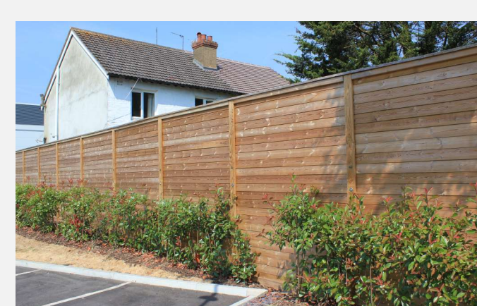
(3) JAKOUSTIC REFLECTIVE (ACOUSTIC) FENCING
