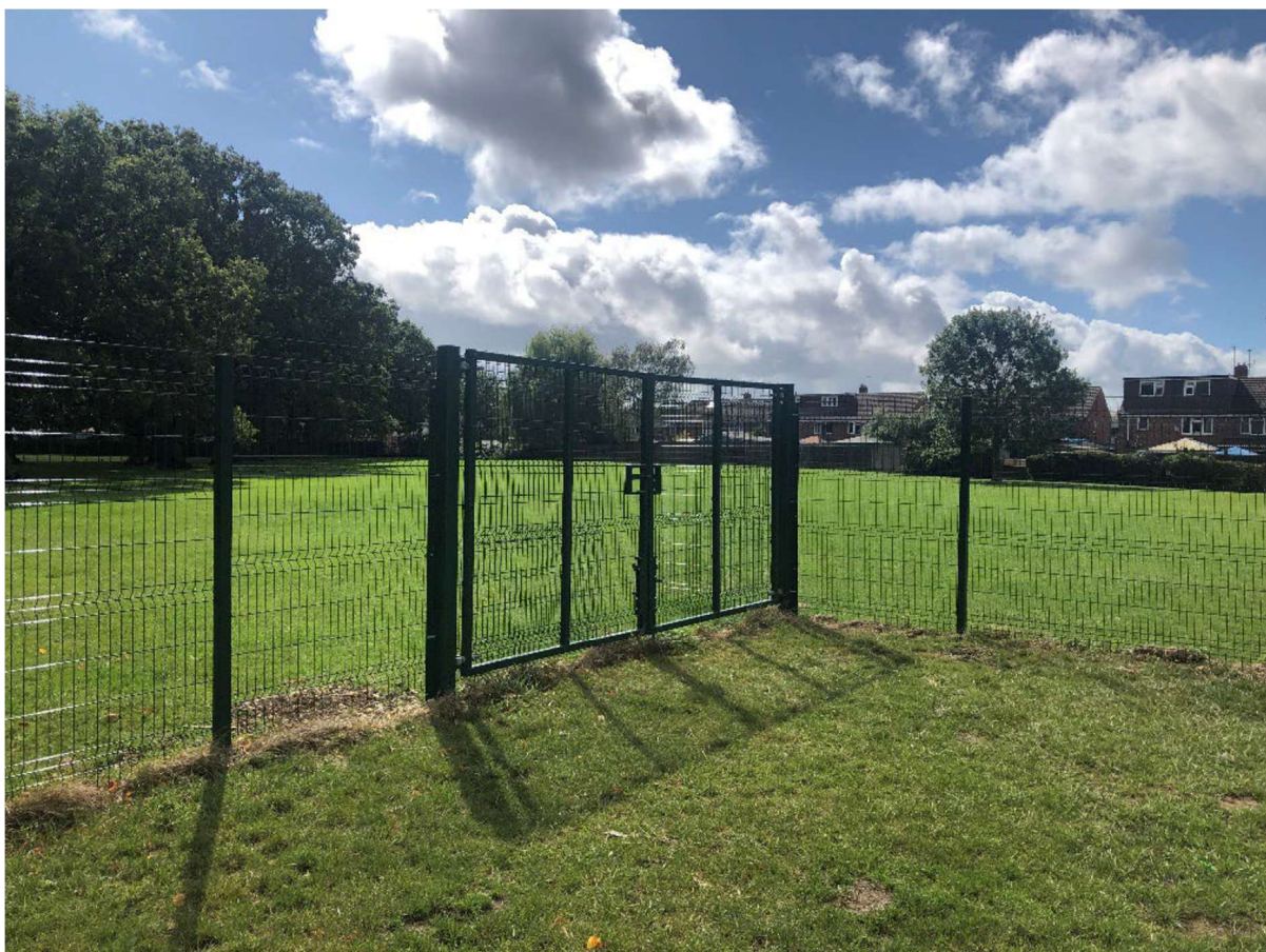
Fig. 4: Existing green PVC-coated welded mesh site fencing, to be made more opaque with additional green netting to screen from park
