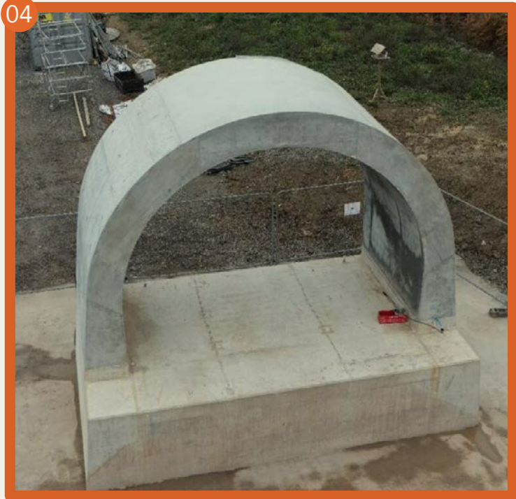
Havant Thicket Reservoir Culvert Section
