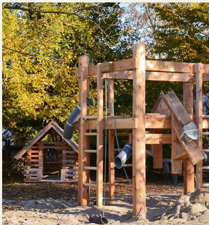
Timberplay Building Site
