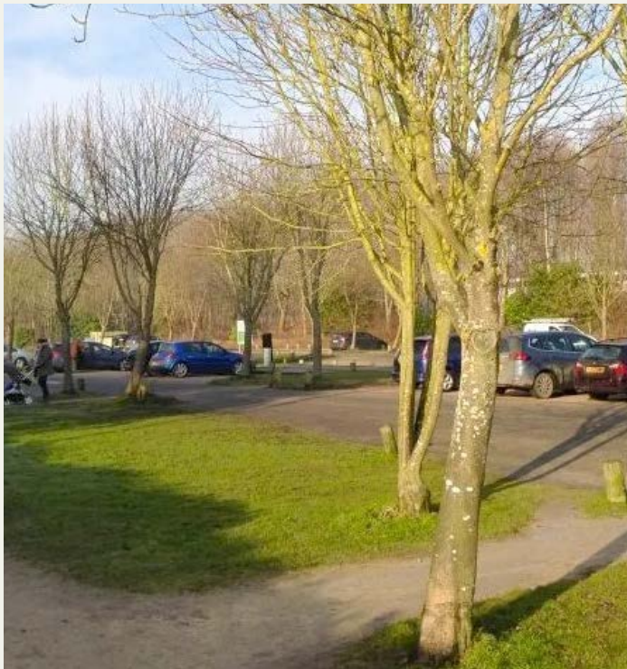
Tarmac broken out for Tree Planting
