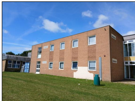
Photo 2 Romsey Block – Eastern elevation
