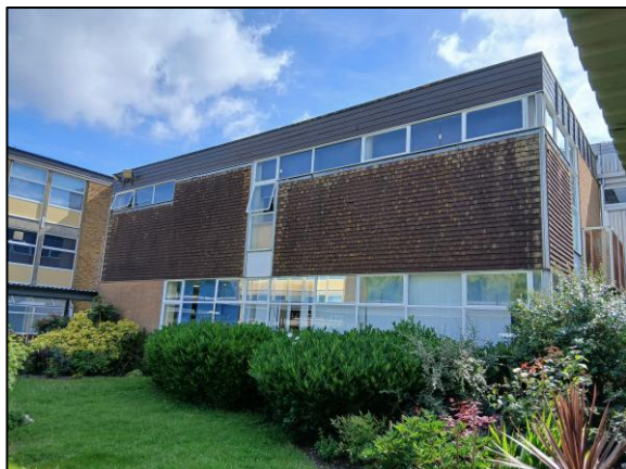
Photo 1 Romsey Block – Western elevation
