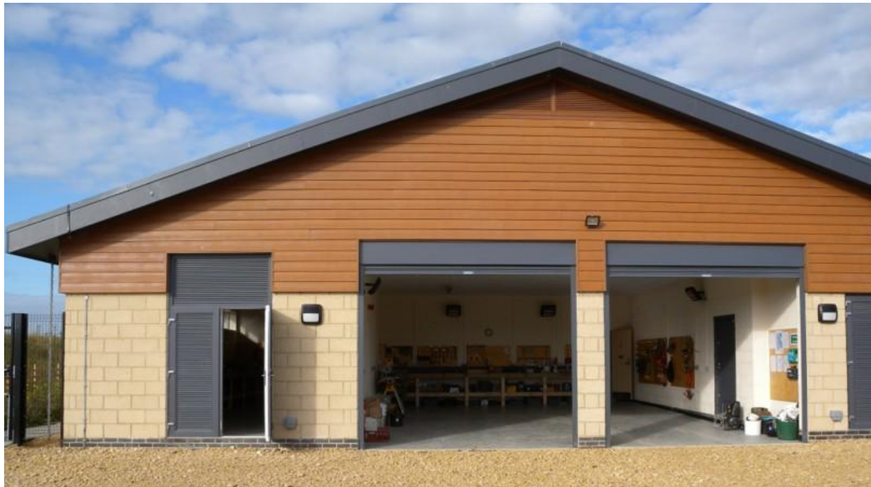
Example of a ground's maintenance store/ workshop at Rutland Water (Anglian Water) with level access and roller shutter doors
