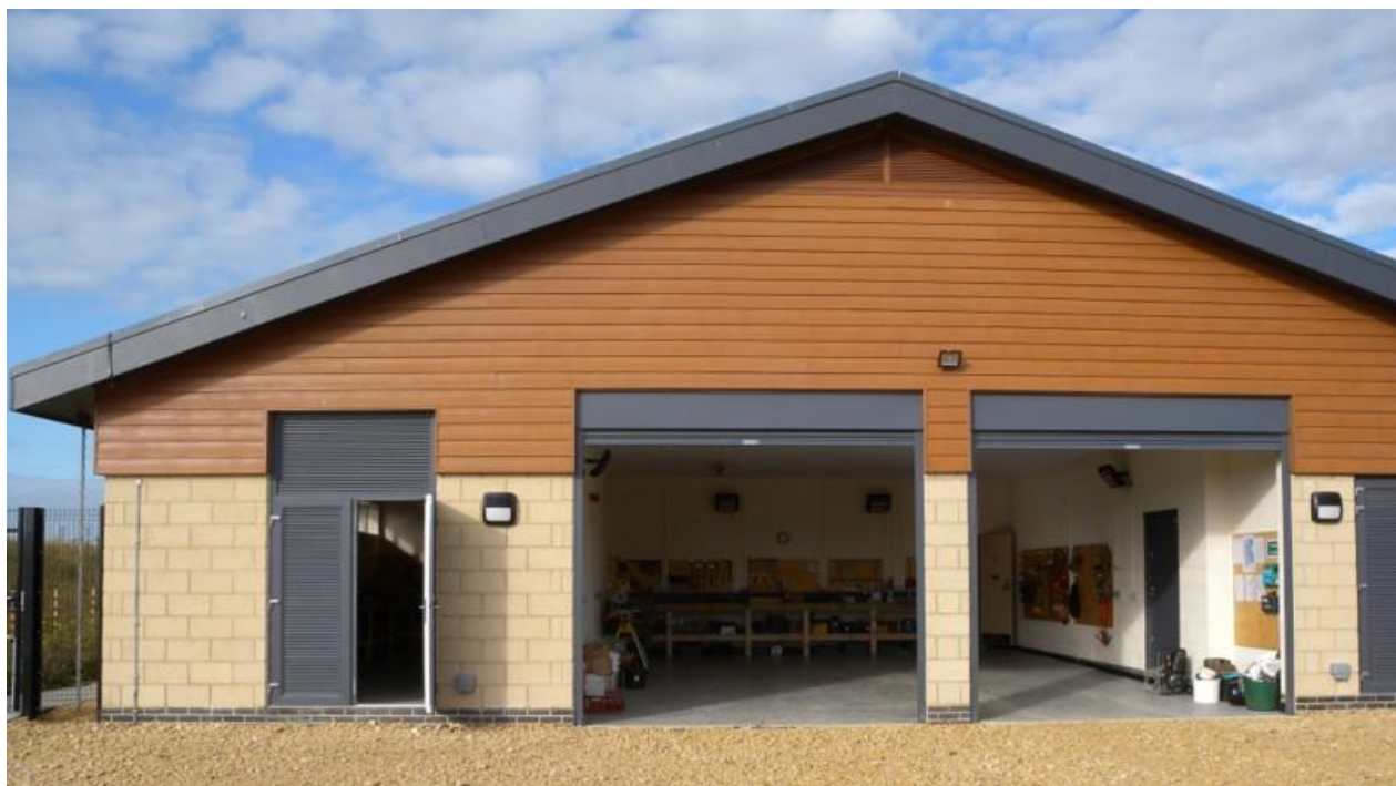
Example of a ground's maintenance store/ workshop at Rutland Water (Anglian Water) with level access and roller shutter doors
