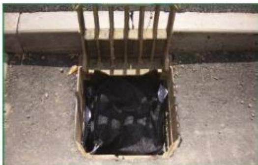
5. Close gully grid.
