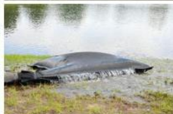
Cut open bag to show trapped silt
