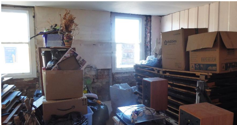
Room awaiting repair
