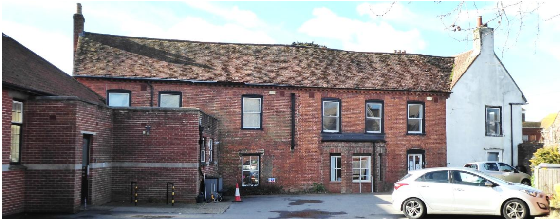
East wing of Church House from Hall car park
