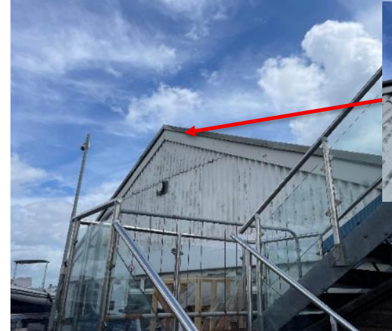
Eastern elevation showing gaps at the base of the roof
