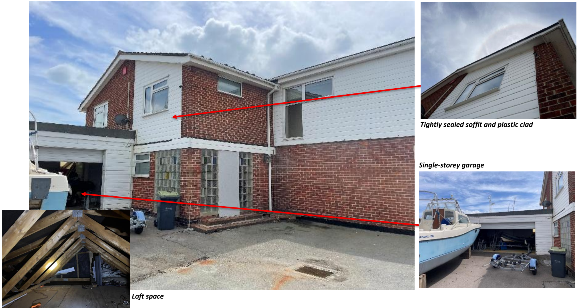
Figure 4. Annotated north-eastern elevation of Building 1 (taken May, 2025).
