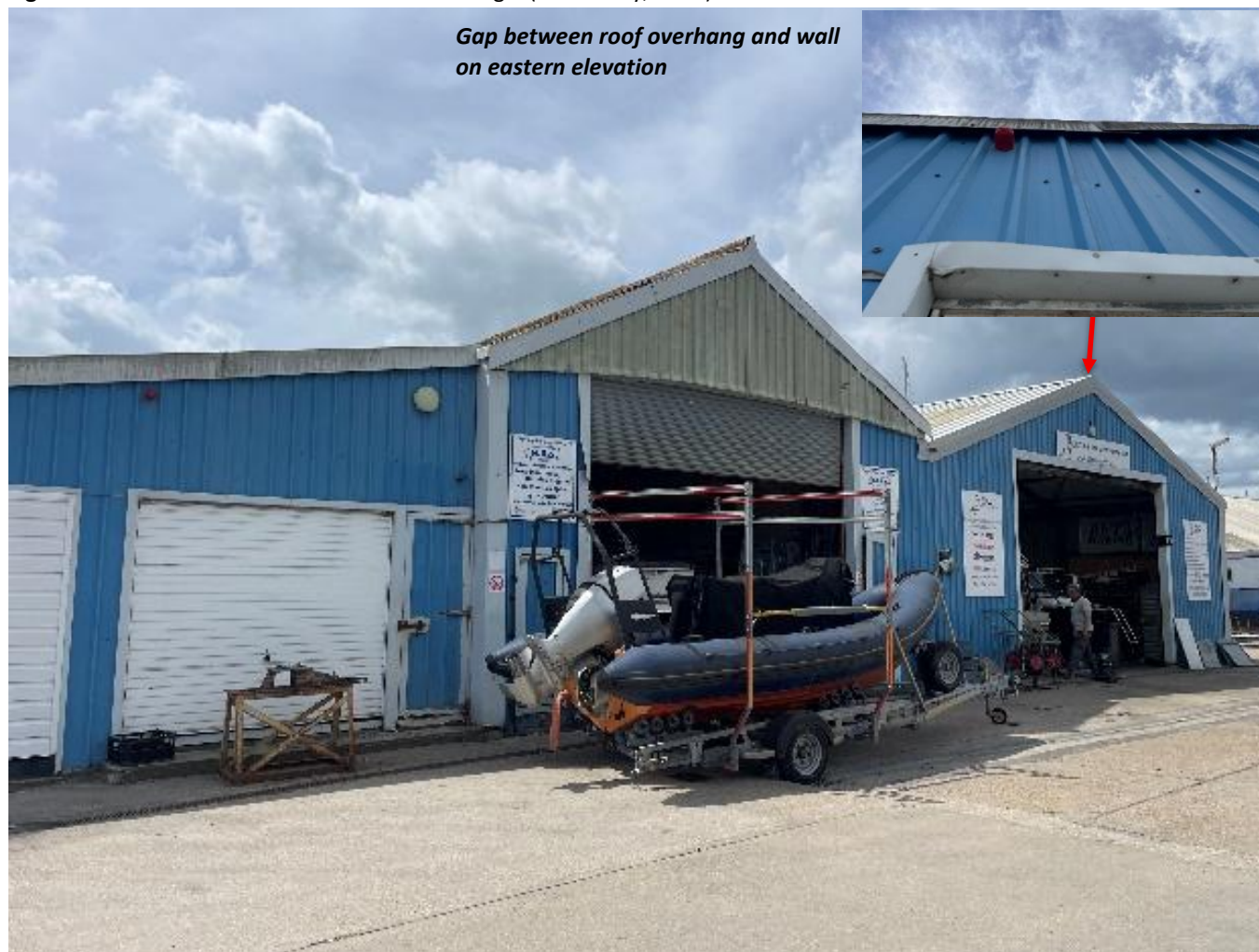
Figure 5. Annotated eastern elevation of Building 2 (taken May, 2025).
