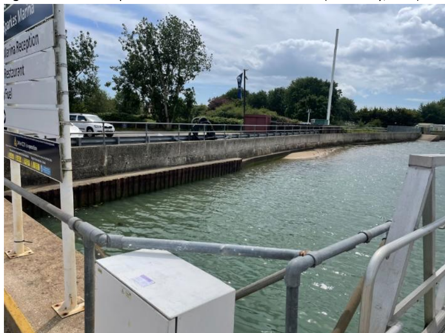
Figure 10. Area of suspected mudflat to the west of the site (taken May, 2025).
