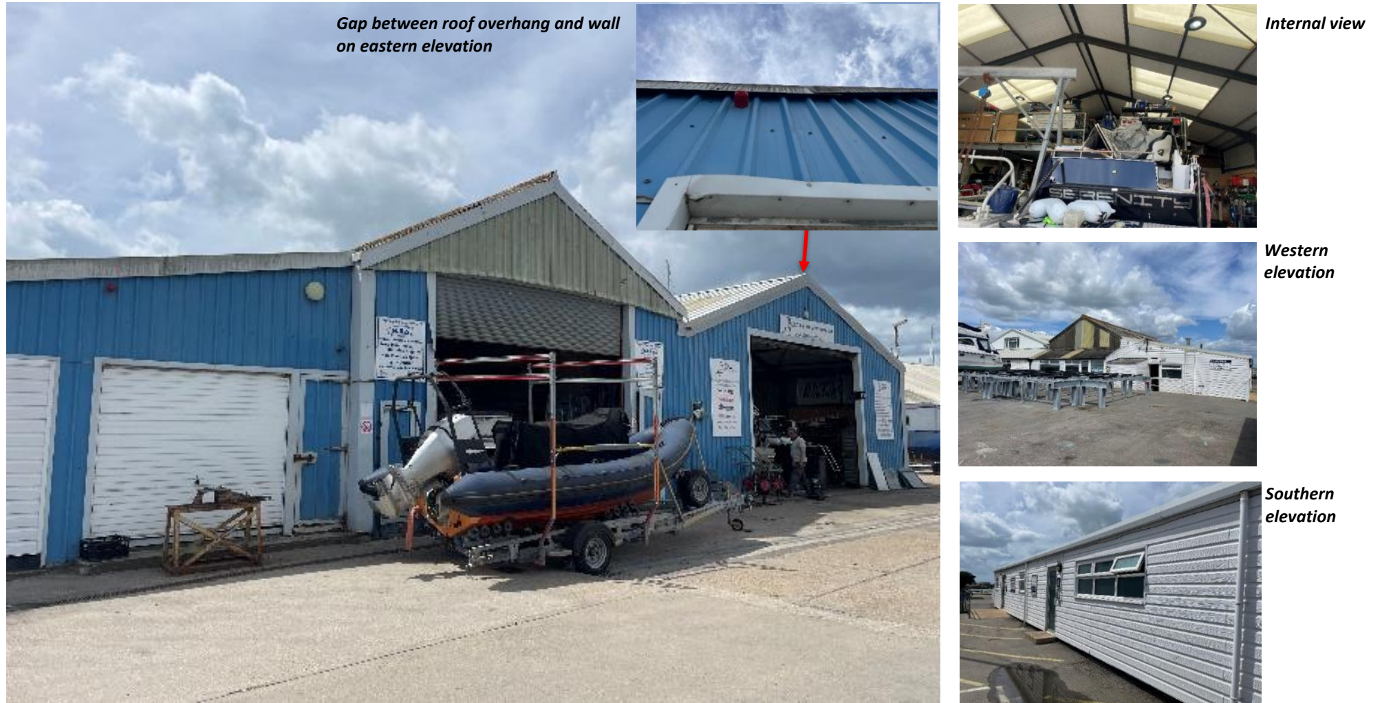
Figure 13. Annotated eastern elevation of Building 2 (taken May, 2025).
