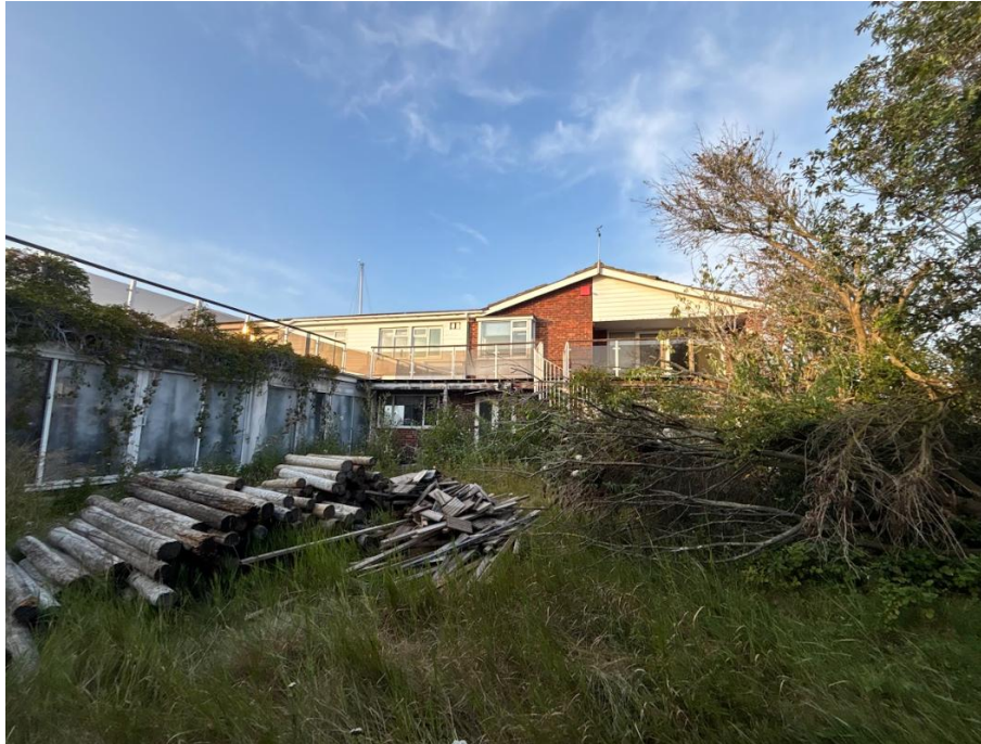
Figure 8. Vegetated garden (u1 - 828) on site (taken July, 2025).
