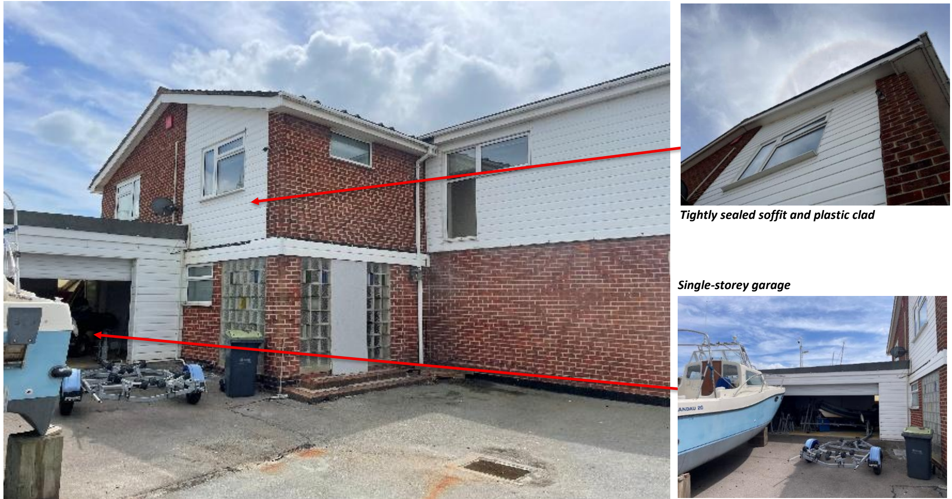
Figure 12. Annotated north-eastern elevation of Building 1 (taken May, 2025).
