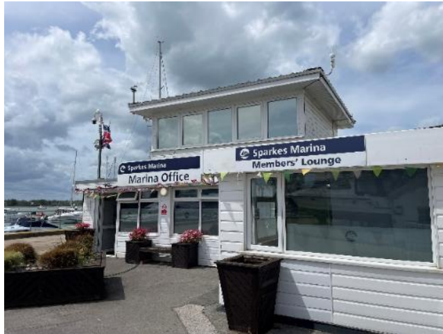
Figure 14. Annotated southern, eastern and northern elevations of Building 3 (taken May, 2025).
