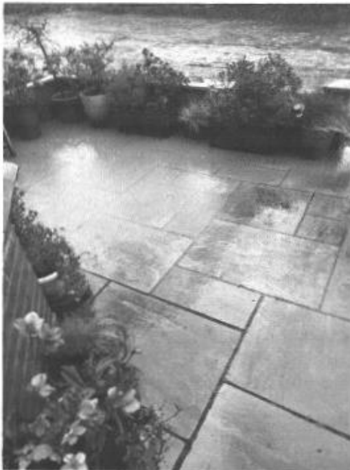
Photo 4: Standing water in my front garden at no.6
