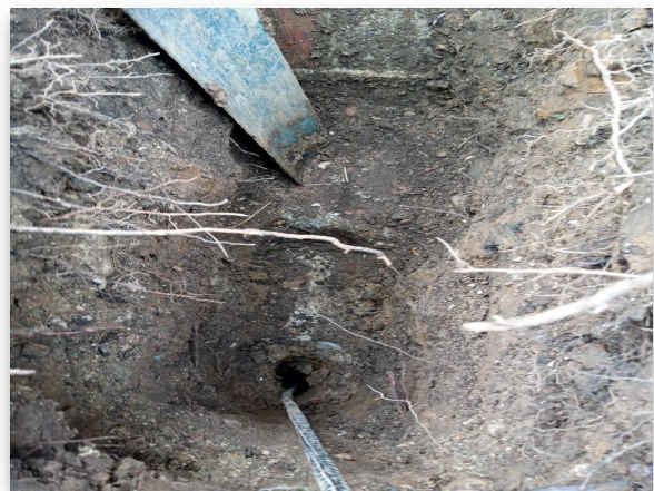
Fig 2.2: Trial Hole 2 Footing
