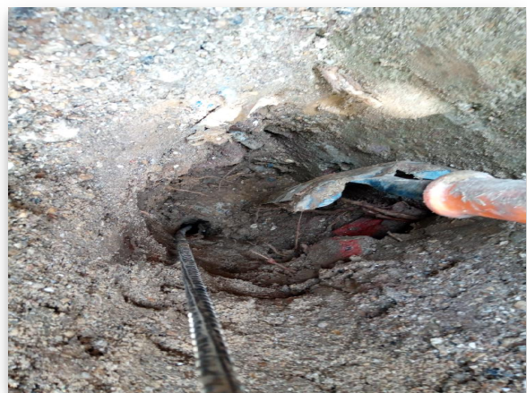
Fig 3.2: Trial Hole 3 Footing
