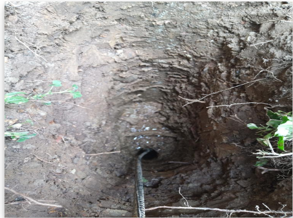
Fig 1.2: Trial Hole 1 Footing
