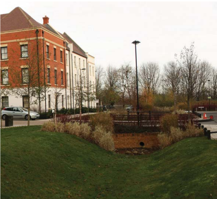
78 | Example of SuDS space and headwall structure as part of an access road. Upton, Northampton
