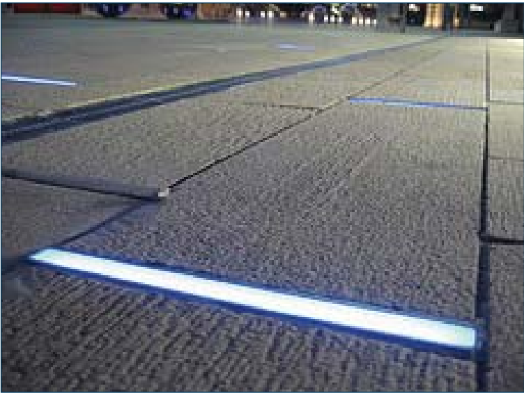
80 | Example of pavement lighting within feature space
