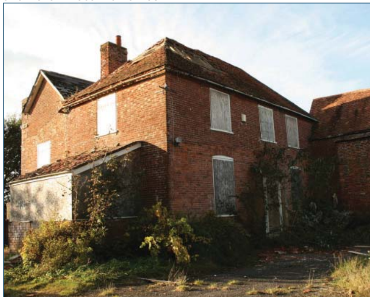
03 | Grade II Listed Farmhouse - Plant Farm
