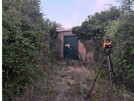
V1 B1-2 surveyor photo
